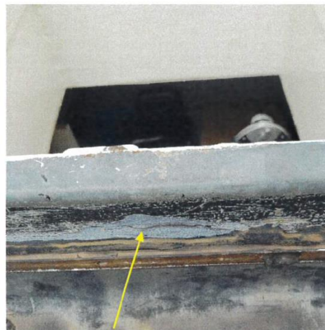
Old flashing mastic present at chimney (top & perimeter), around access hatch and perimeter of roof
