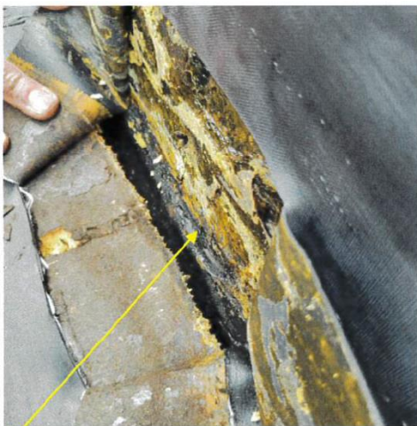
Old flashing mastic present at chimney (top & perimeter), around access hatch and perimeter of roof
